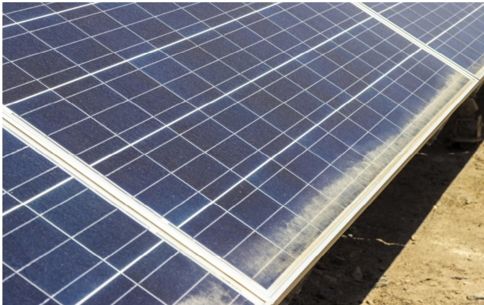
Picture 2: Dusty surface of a solar cell illustrating the need for a good cleaning mechanism to maintain efficiency.
